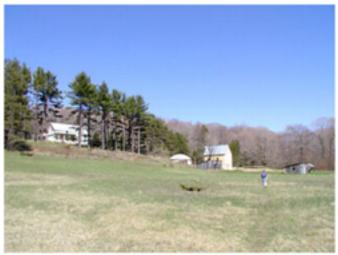
Family home is to the left, Barn to the right. Note the interesting round structure just to the left of the barn. It was built by pouring concrete walls, filling the building with dirt and rocks by hand and then pouring cement atop the soil.
